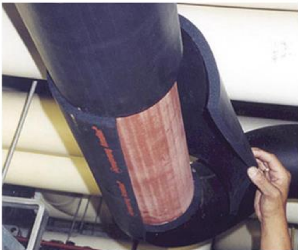
No corrosion even after 25 years. Armaflex installation at Rabo Bank, Amsterdam.
